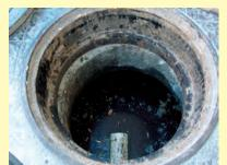
No Outlet T installed Allows FOG to be discharged which causes sewer blockages.
