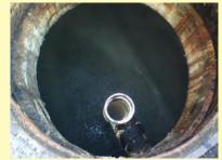
**Proper Outlet T installation**PVC schedule 40, to within 12" of the tank bottom prevents FOG discharge.
