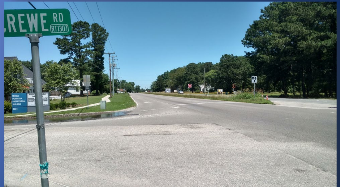
Intersection of Crewe Road and US 17
