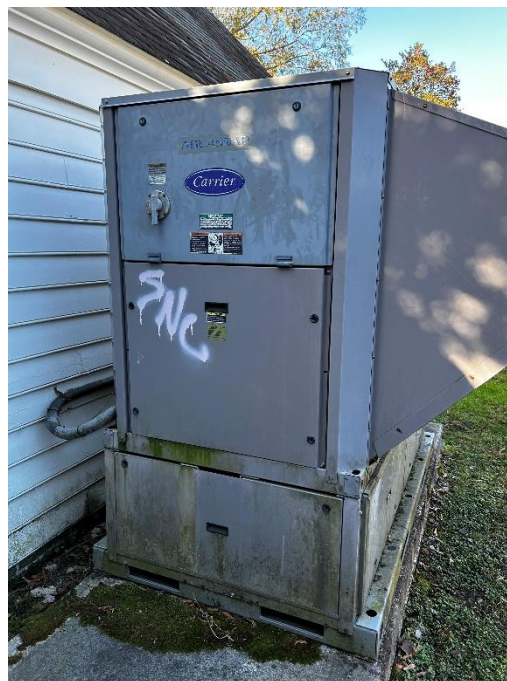
Air-cooled, direct-expansion chiller
