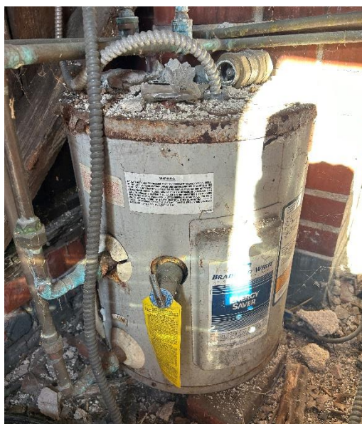
Electric tank water heater
