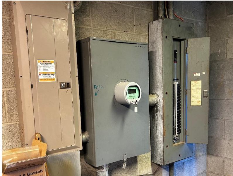
120/208V, 3Ø, 4 Wire 320 Amp electrical service in rear building utility room
