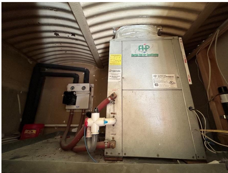
Water-source heat pump
