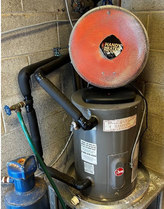
Electric tank water heater located in the main utility room
