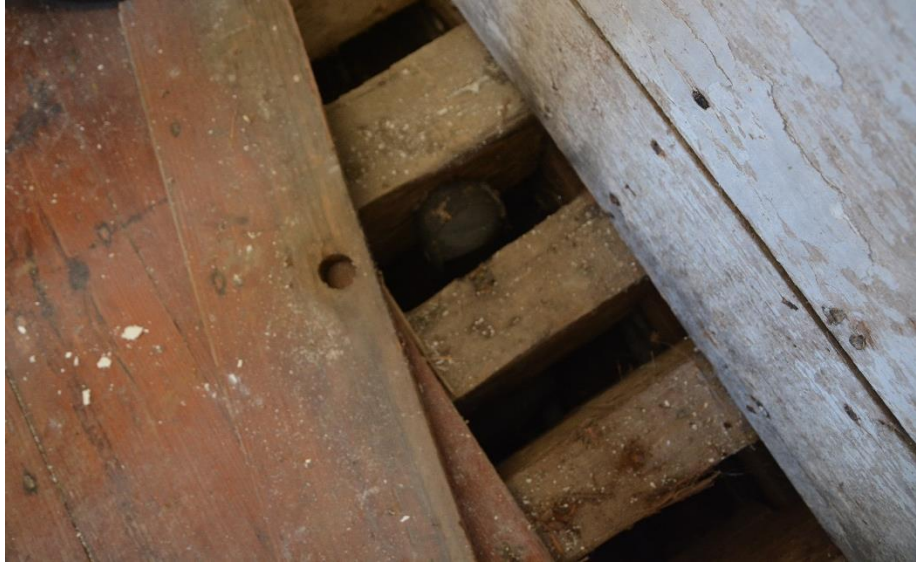
Floor structure at wall.
