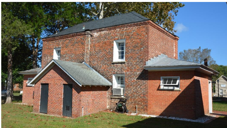
View of rear of Old Jail showing all three roofing types
