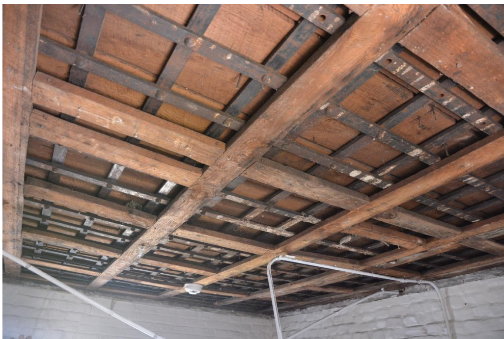
Iron bar lattice in ceiling in second-floor west room
