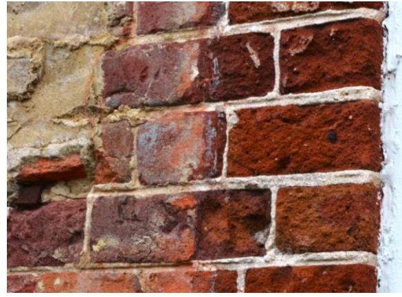
North wall sandblasting damage.
