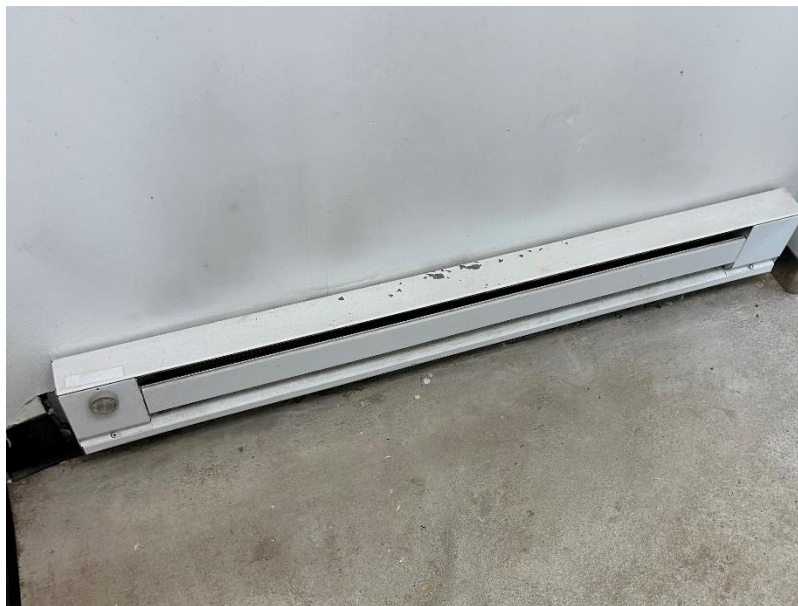
Electric baseboard heaters in restrooms
