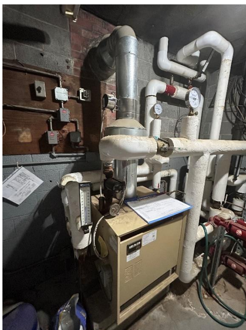
Hot water boiler
