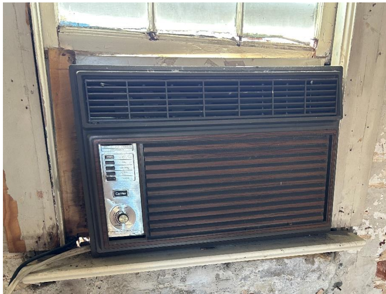
Window terminal units (packaged units)
