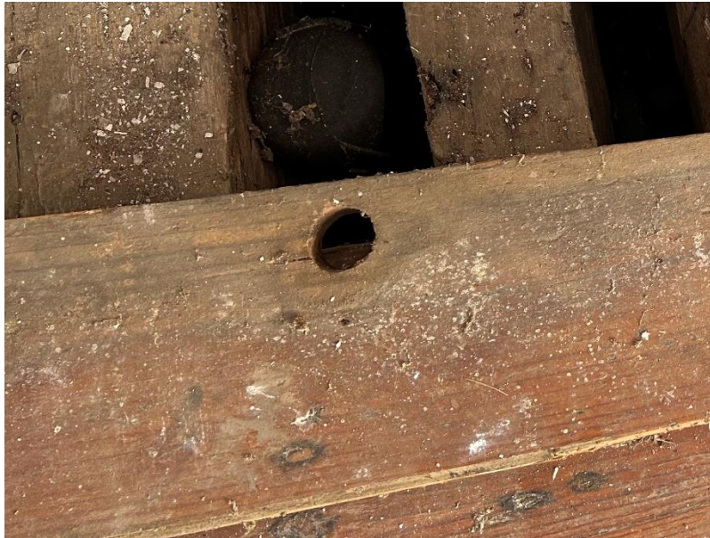
Possible radiator piping hole at floor
