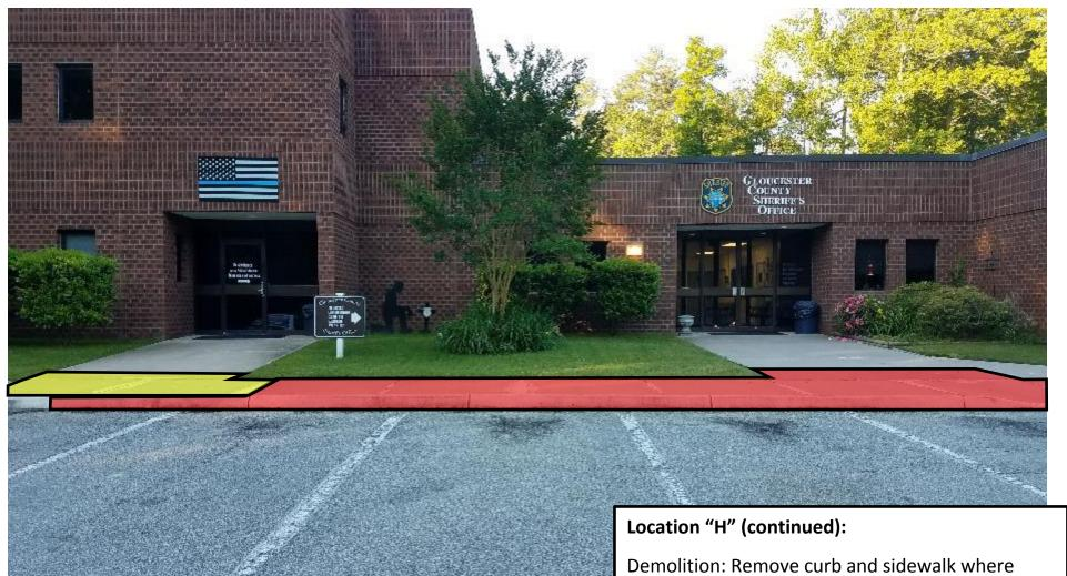
Demolition: Remove curb and sidewalk where shown in red. Remove sidewalk where shown yellow.
