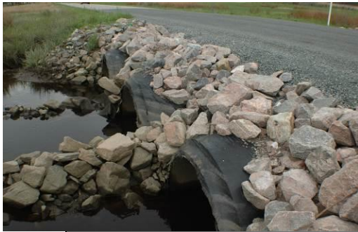
Figure 15: Roadside Ditch in the Southeastern Portion of the County.
